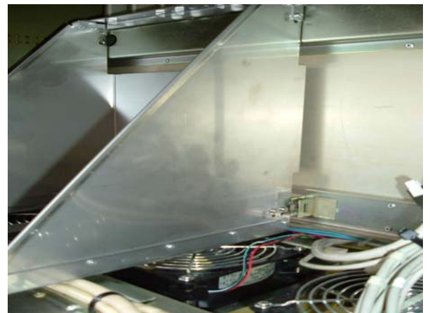
AM35 mounting frame installed
