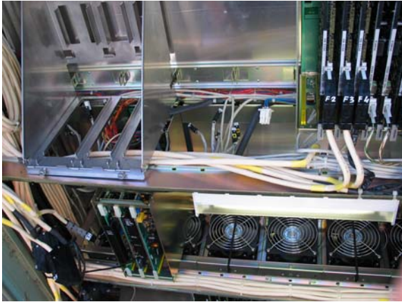
Mounting frame shown installed. Existing RIM cables are tied behind the cable tray and beneath the AM35 mounting frame.
